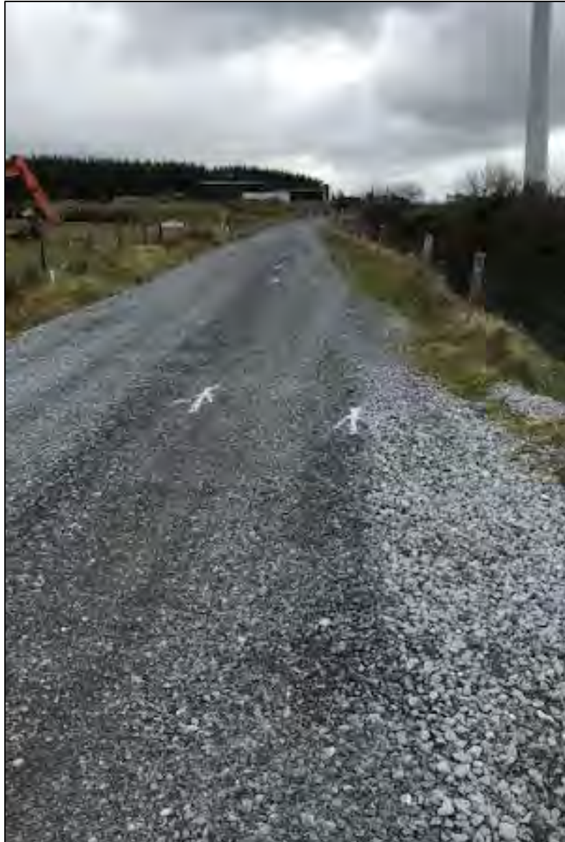
Figure 3.6: Typical Access Track
