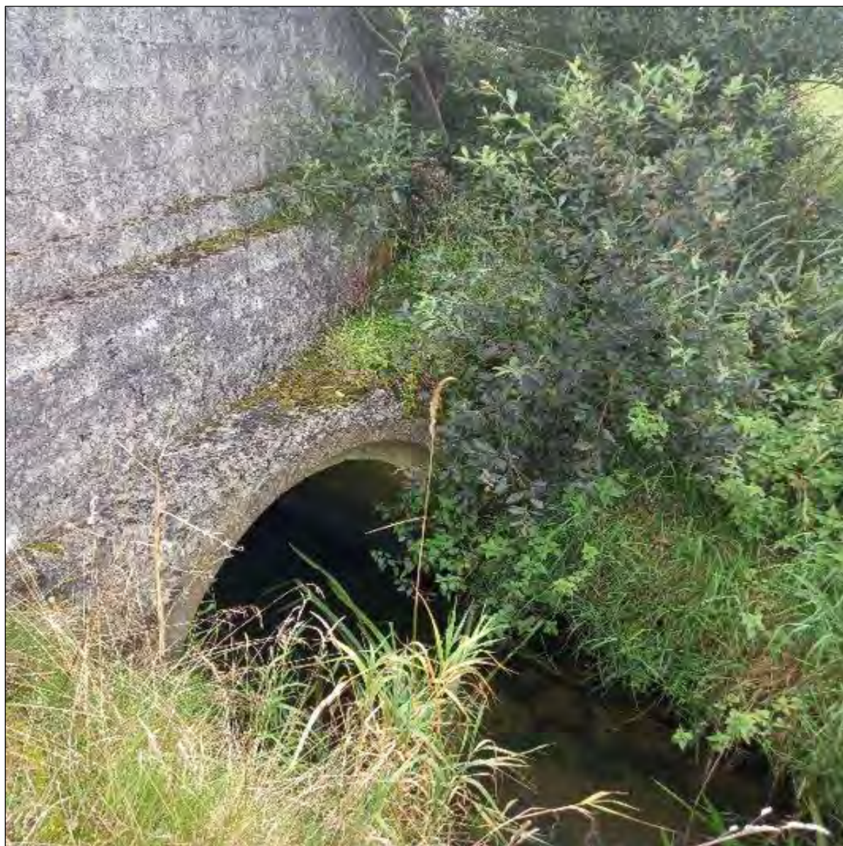
Plate 10.4: Watercourse crossing, looking north west
