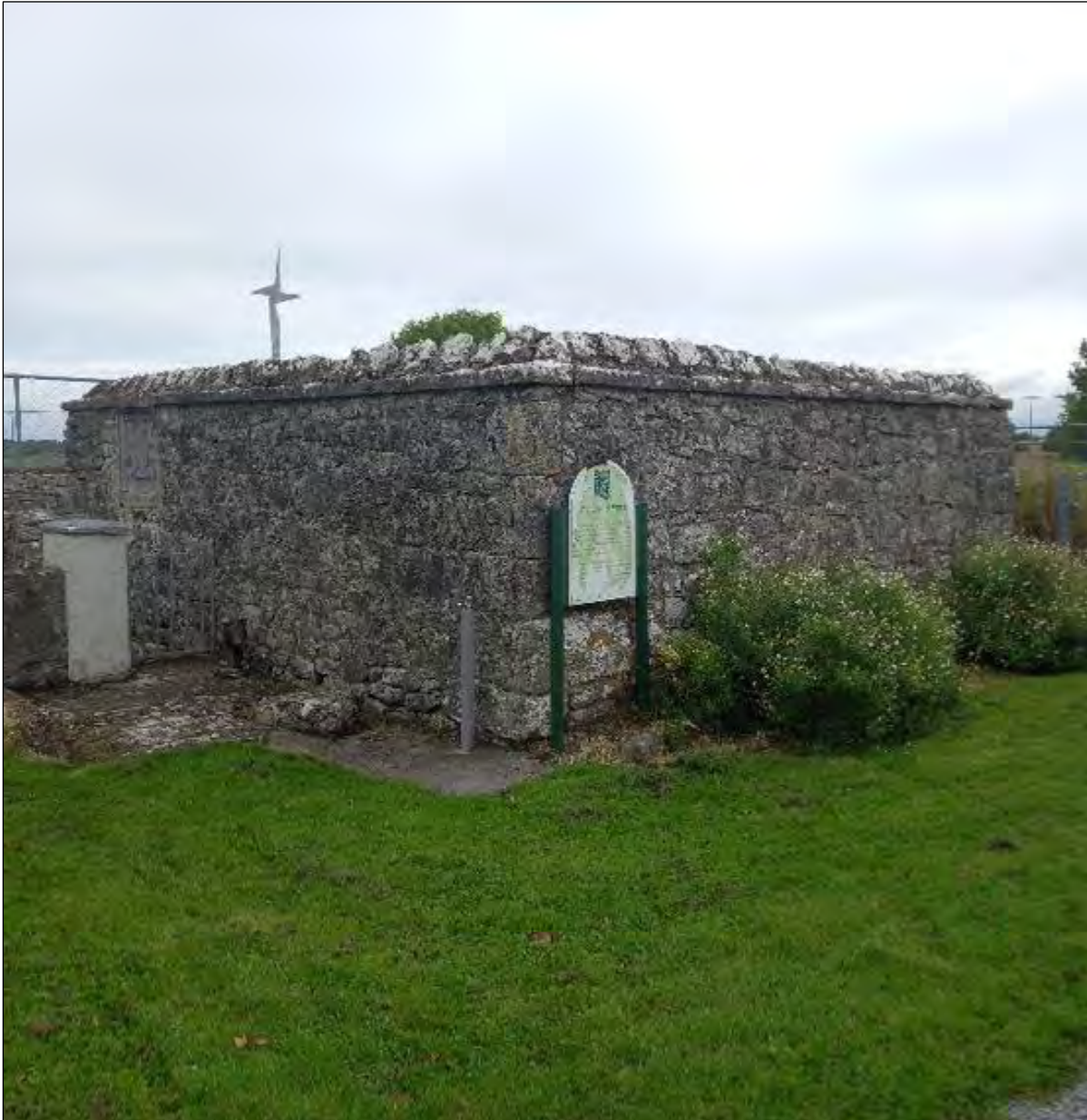
Plate 10.6: Building (RMP RO048-108002 bath house), containing RMP RO048-108003 (armorial plaque) and RMP RO048-108005 (stoup), looking east
