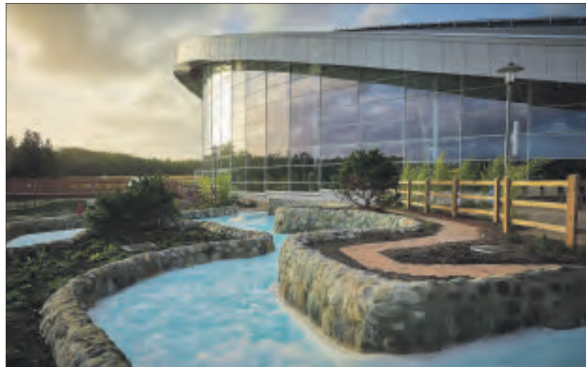
The 'subtropical swimming paradise' at Center Parcs Longford Forest is to be extended as part of a €100 million expansion of the resort which will get underway in September.
